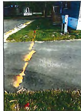
Private utilities marked or flagged.
