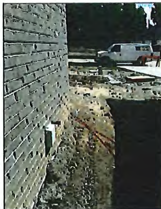
Clear pathway from meter location to street.
